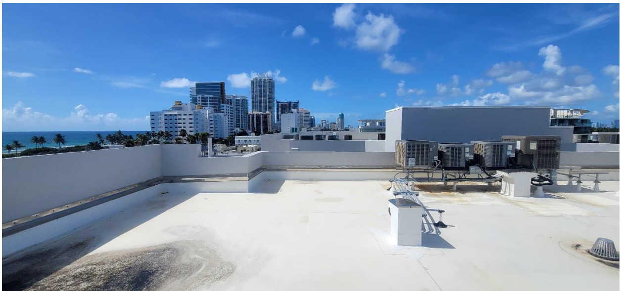
Photo #30 - Northeast Corner
