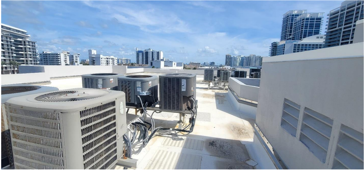
Photo #25 - West Side – Center Section
