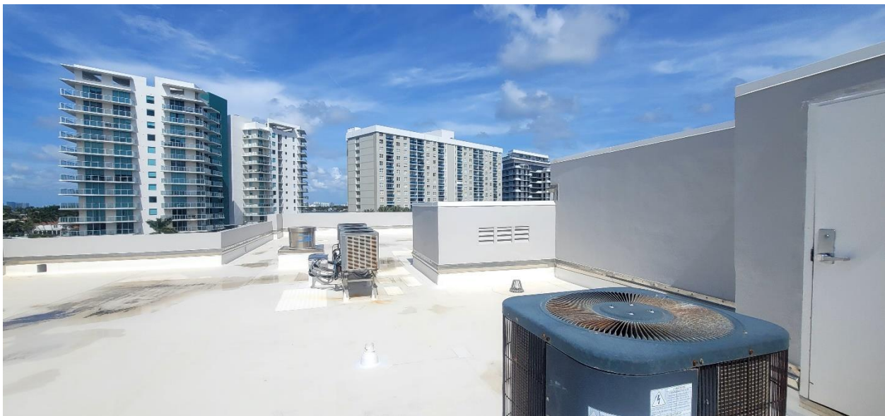
Photo #24 - South Side – Center Section
