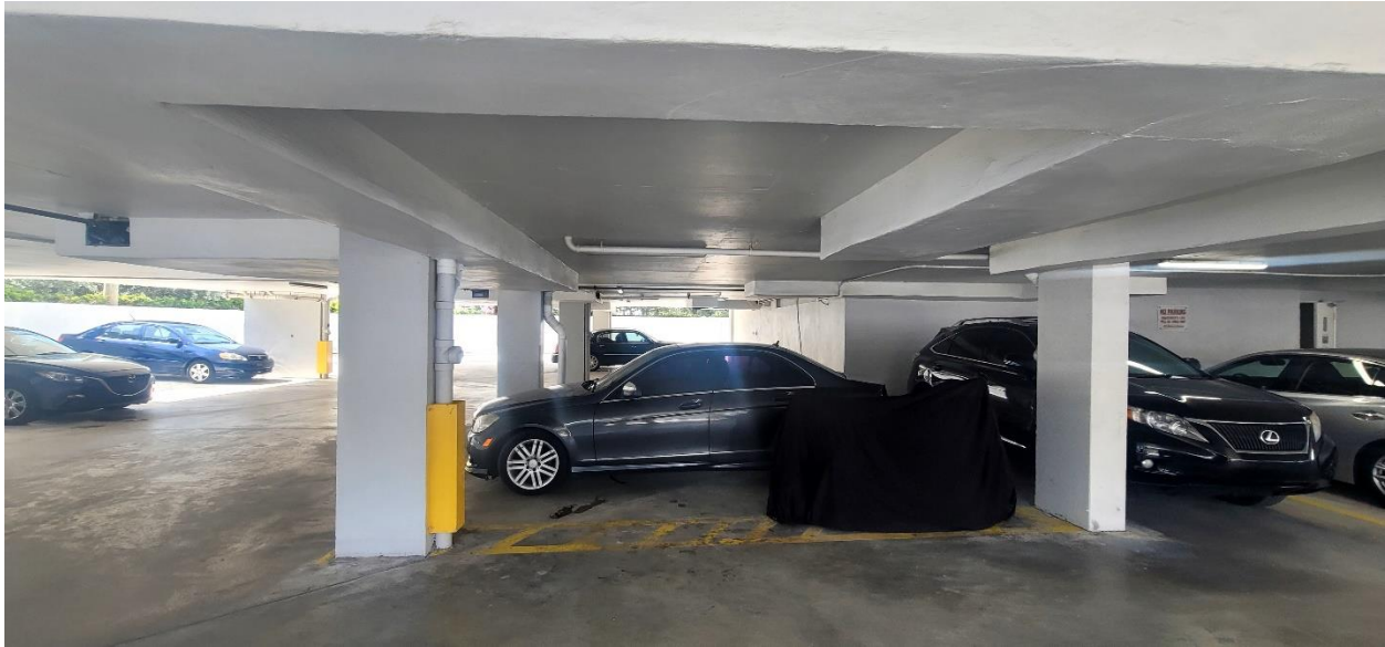
Photo #39 - Northeast Corner
