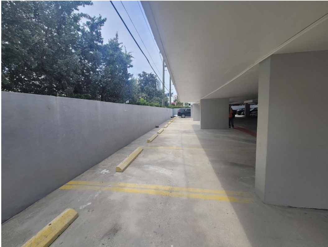
Photo #5 – Freshly Painted and Waterproofed, Fully Repaired Balcony Underside
