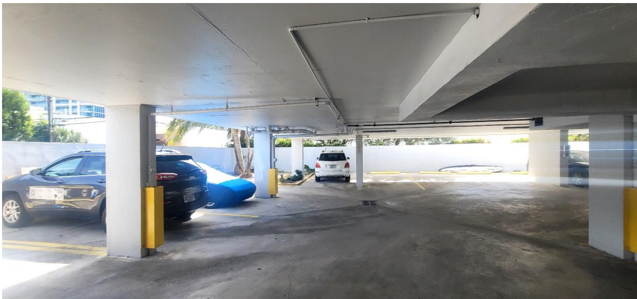
Photo #38 - North Side – East Section
