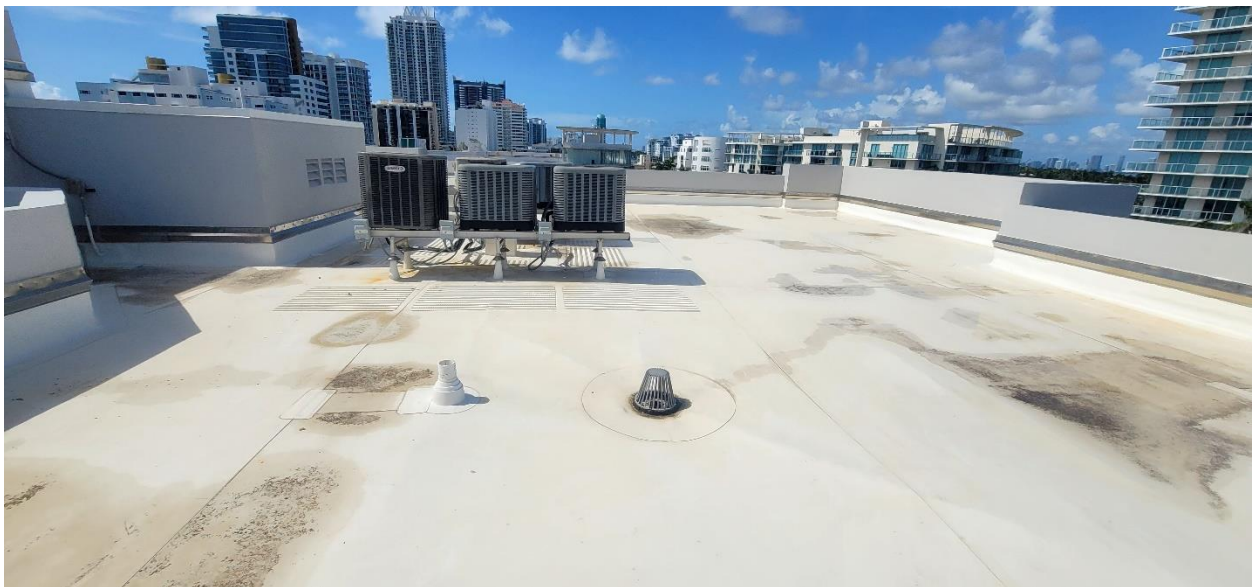
Photo #34 - West Side - North Section
