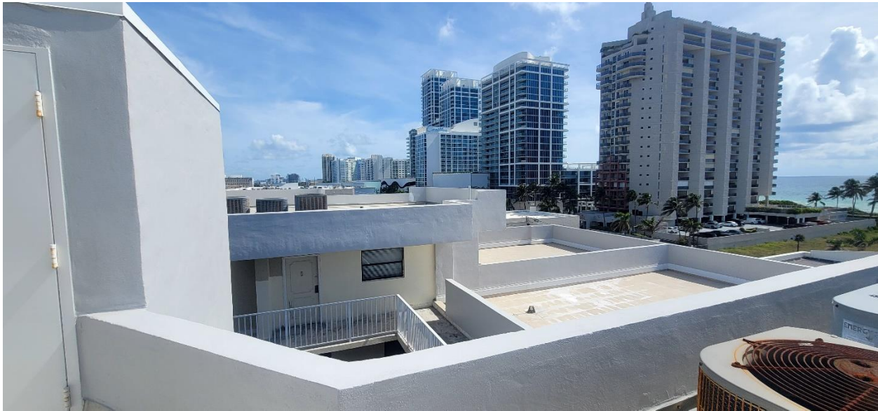
Photo #23 - South Side – Center Section
