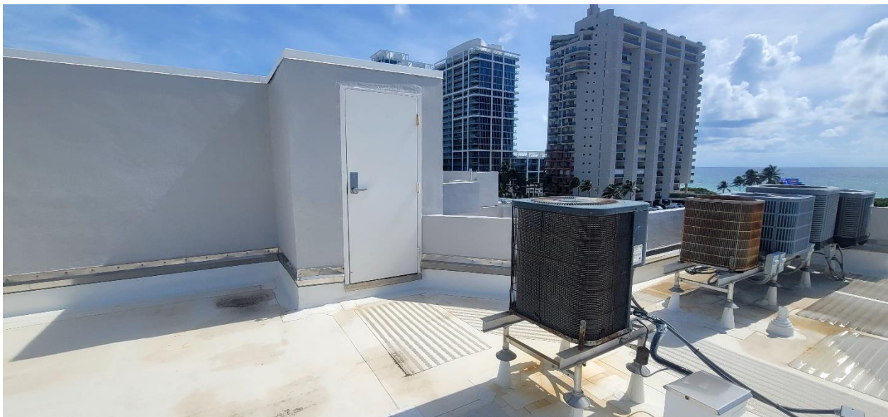
Photo #22 - South Side – Center Section
