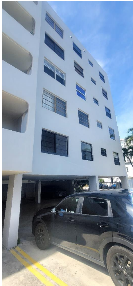
Photo #20 - North Elevation – West Section
