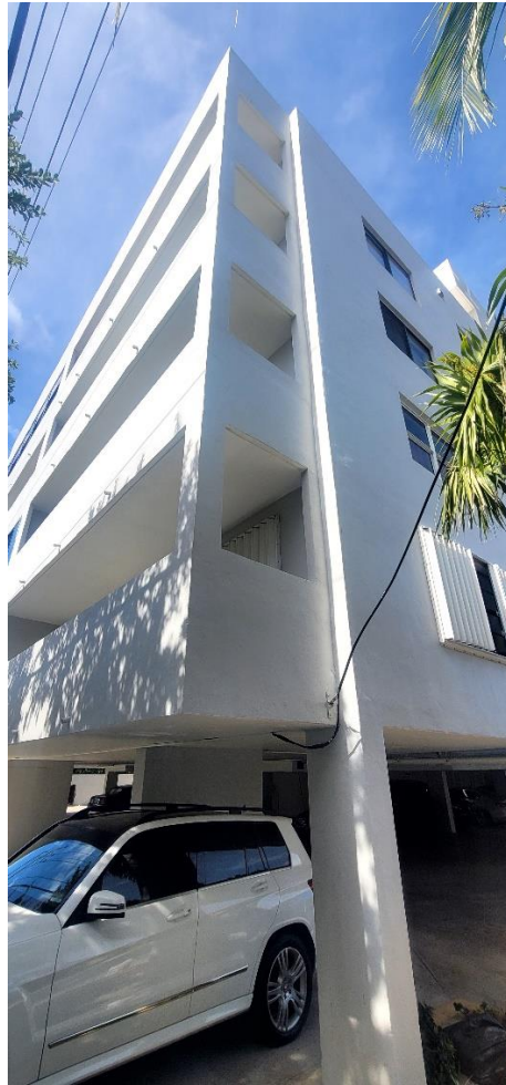
Photo #15 - Northeast Corner
