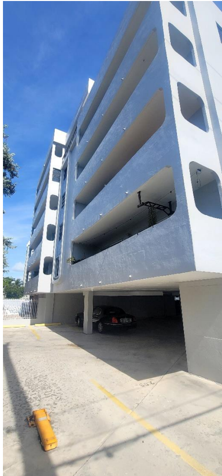
Photo #11 - South Elevation – East Section
