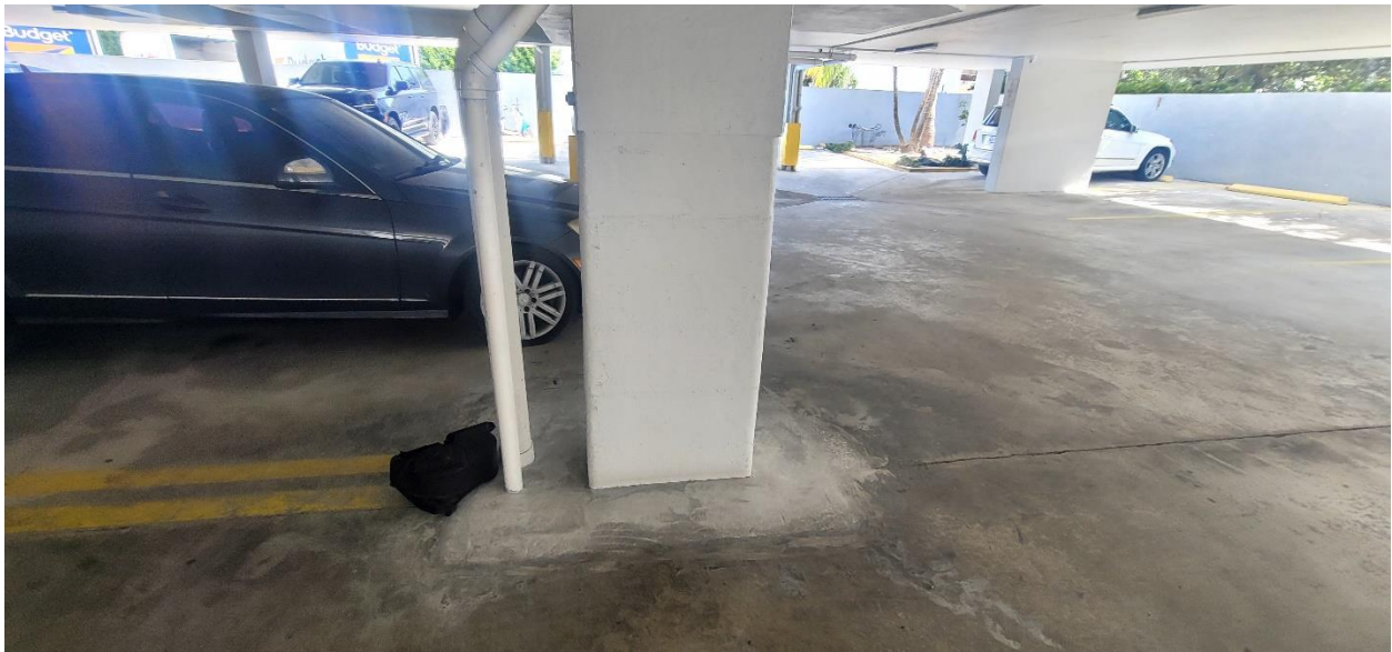
Photo #42 - Southeast Corner
