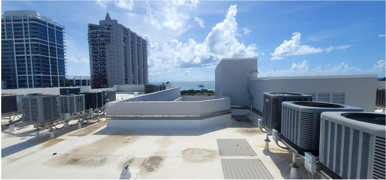
Photo #27 - West Side – Center Section
