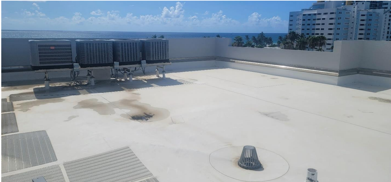
Photo #21 - South Side – Center Section
