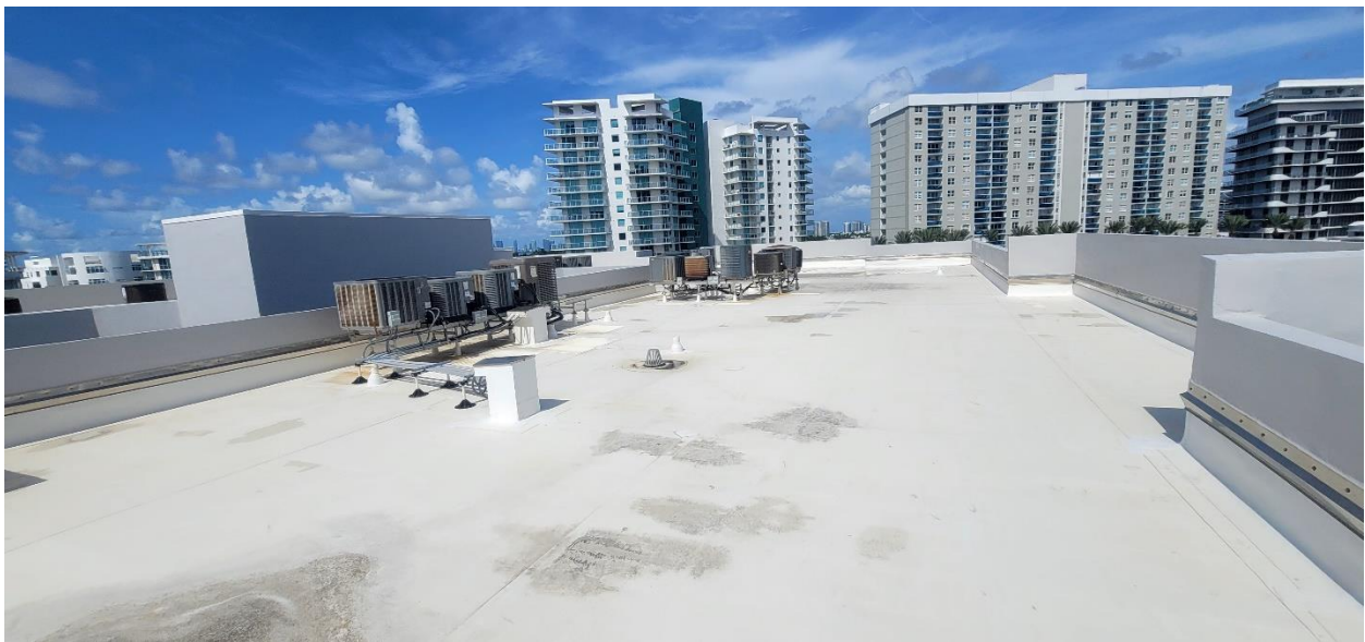
Photo #32 - North Side - Center Section
