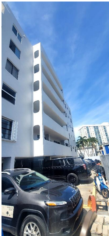
Photo #18 - North Elevation – Center Section
