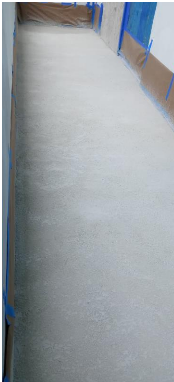
Photo #6 – Freshly Waterproofed Balcony Deck Surface
