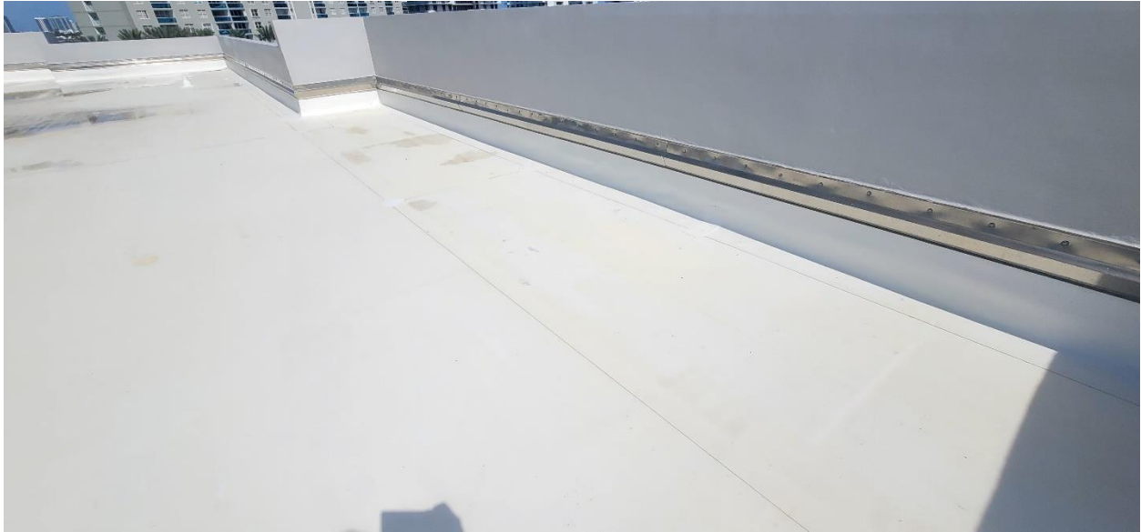
Photo #33 - North Side (Wall)
