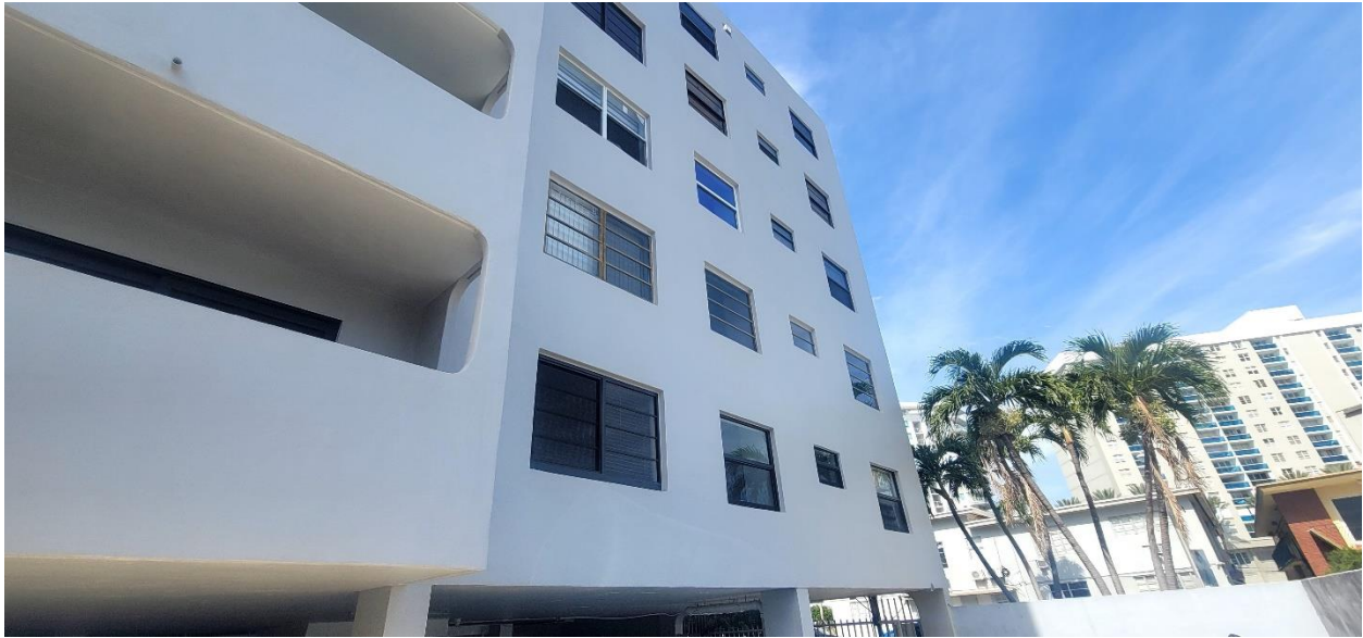
Photo #19 - North Elevation – West Section
