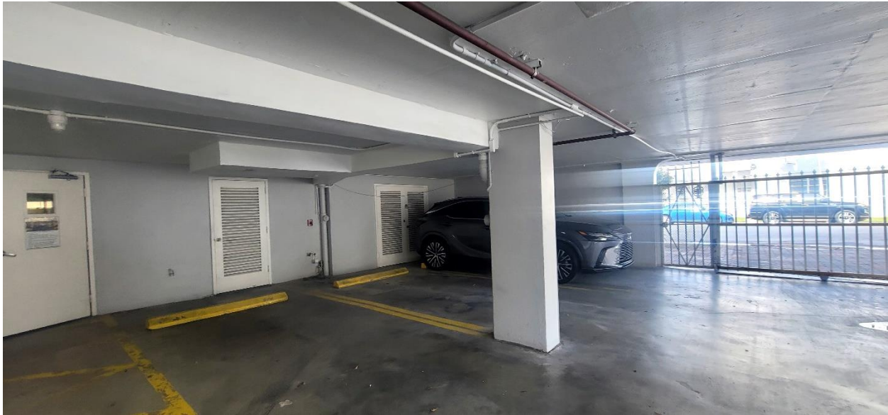
Photo #35 - West Side – Center Section
