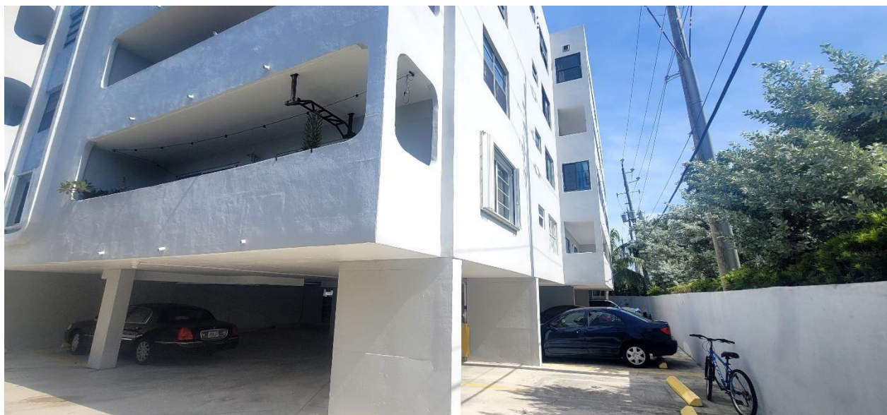
Photo #12 - Southeast Corner
