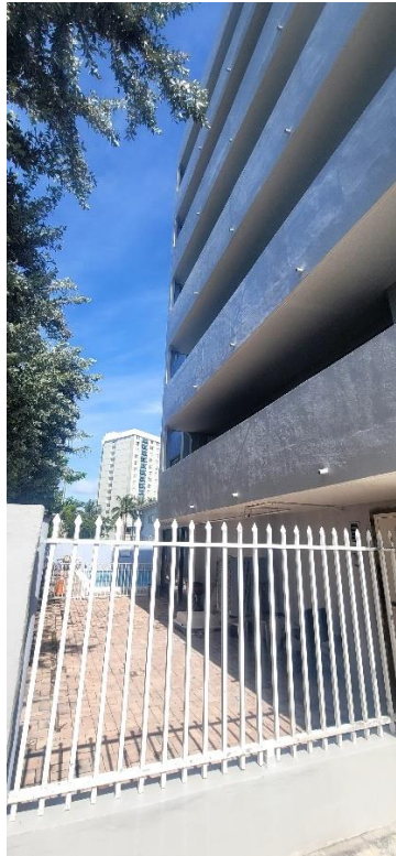
Photo #9 - South Elevation – Center Section
