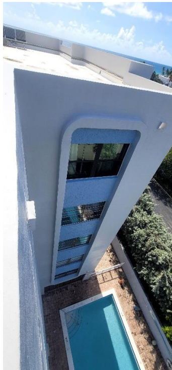
Photo #44 - Window Wall - Adjacent to the Pool
