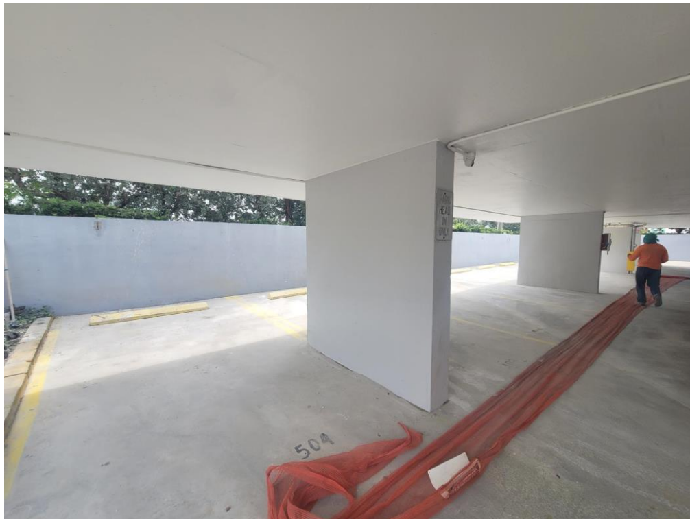
Photo #4 – Freshly Painted Covered First Floor Parking Under the Building
