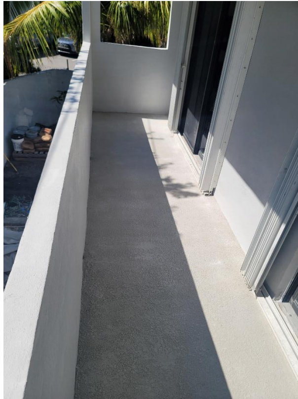
Photo #3 – Freshly Painted and Waterproofed, Recently Repaired Balcony
